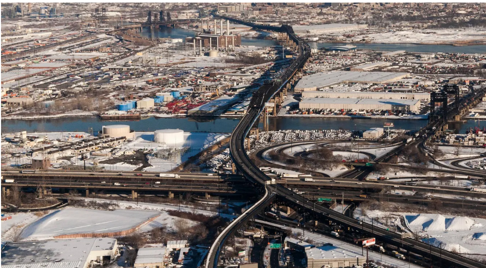
Pulaski Skyway Rehabilitation, NJ
