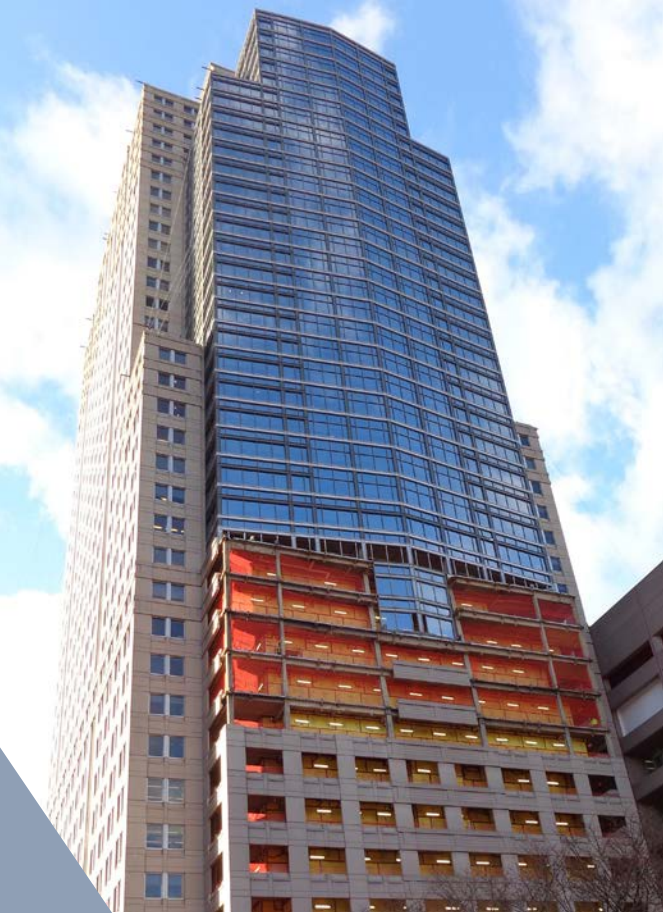
CitiGroup iDAS Installation, New York, NY
