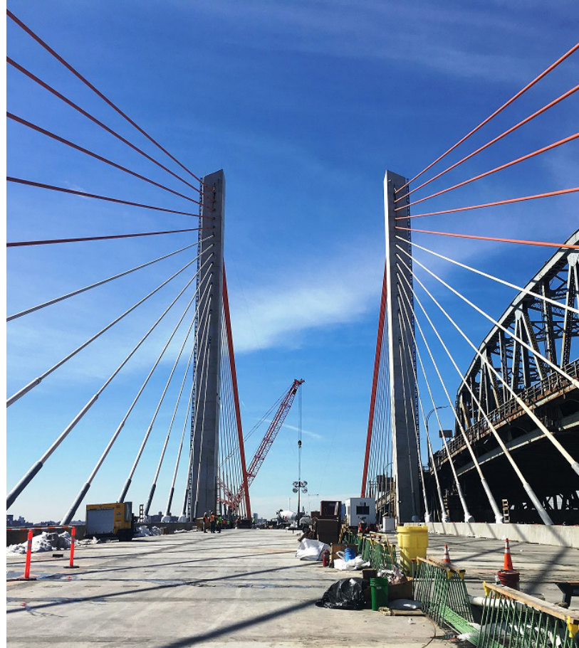
Kosciuszko Bridge over Newtown Creek, Brooklyn, NY
