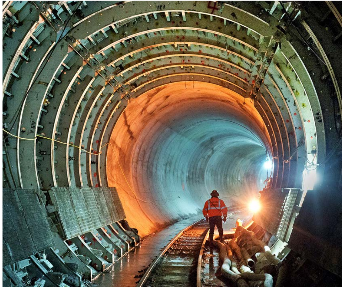
MTA East Side Access, New York, NY
