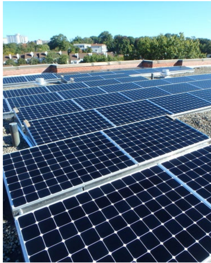
Mapleview Towers Ballasted Solar System Installation, Stamford, CT
